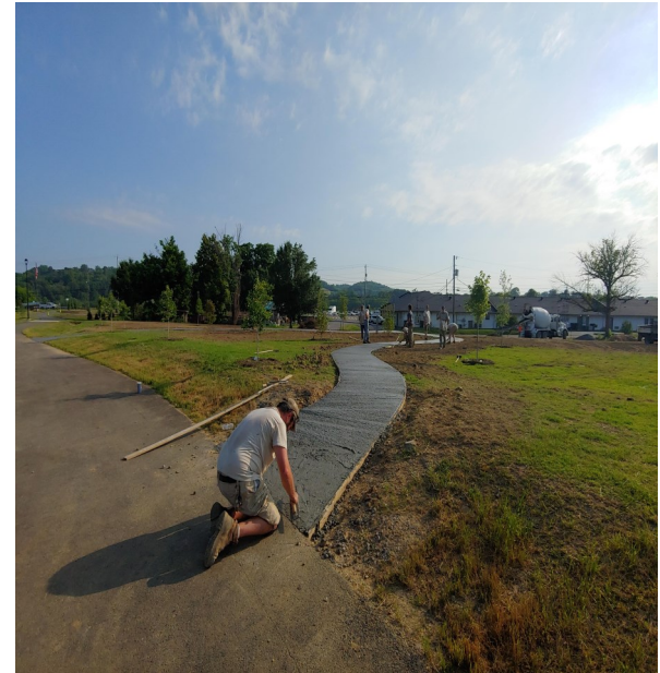
Hal Watson Jr. along with others pour concrete..
