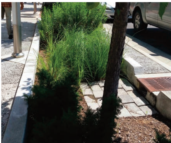
Figure 2: Street side planter boxes. runoff enters the planter boxes through curb cuts (Source: The SMART Center).
