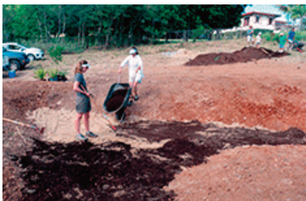
Figure 5.2: Soil amended with compost (Source: USDA NRCS).
