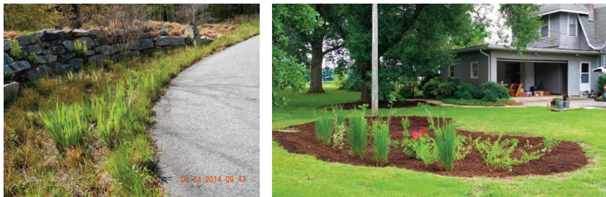
Figure 3.11: Photographs of lot scale runoff reduction measures. Left: a roadside vegetated verge (ie. no curb or gutter) that accepts roadway runoff, uses engineered soils to infiltrate runoff, and conveys excess runoff to a small treatment wetland. Right: a residential rain garden captures and infiltrates runoff from half of the house rooftop and driveway.
