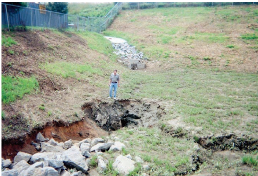
Figure: 7.1 Sinkhole Collapse in SCM.
