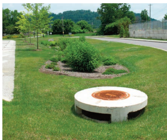
Figure 9: bioretention to capture runoff from a parking lot in Powell TN (Source: The SMART Center).
