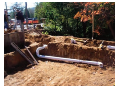
Figure 21: Installation of upturned underdrain and observation well (NC 2012, p:27).
