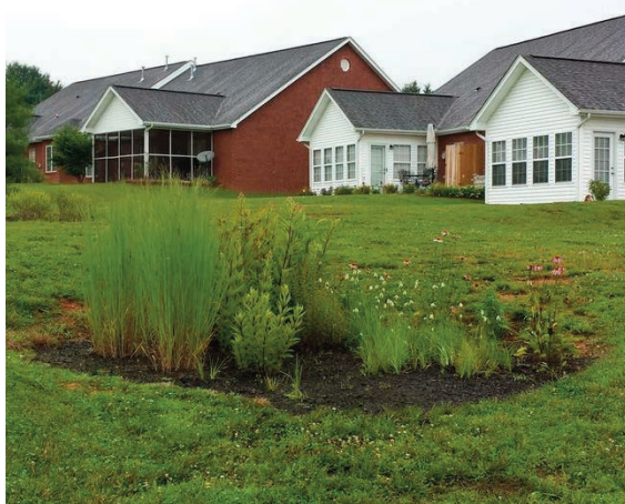
Figure 8: bioretention to capture sheet flow from neighborhood in Knoxville TN (Source: The SMART Center).
