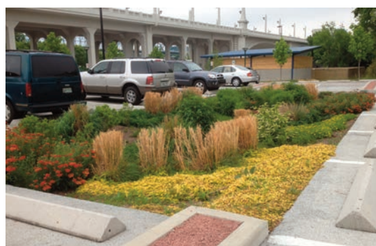
Figures 2 & 3: roof leaders are directly connected to the bed. Bioretention that manages runoff from a parking lot (Source: The SMART Center).
