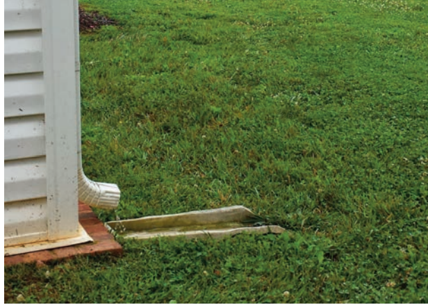
Figure 1: Roof downspout is directed to an infiltration area (Source: The SMART Center).
