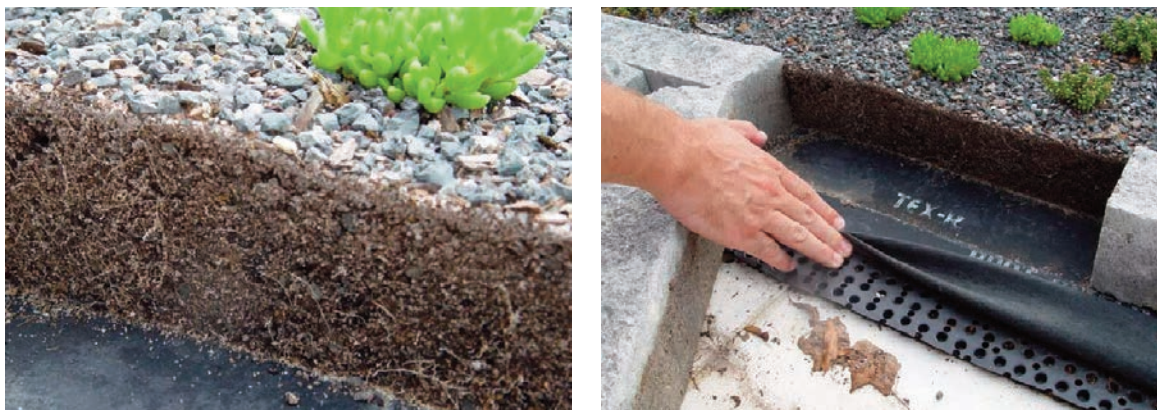
Figure 4: Vegetated roof cross-section (Source: NCSU-BAE).
