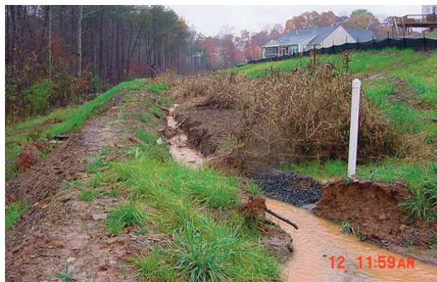
Bioretention swale, installed too early during active construction, has become clogged with sediment.
