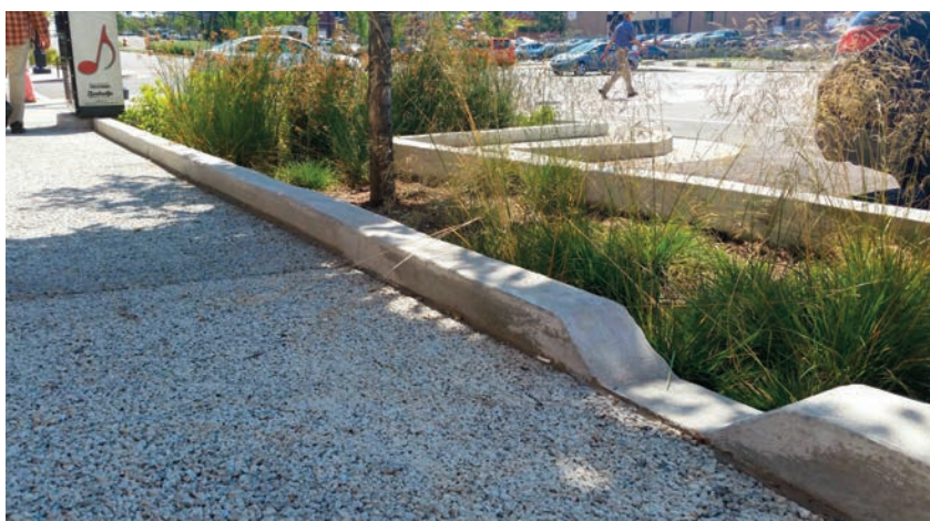
Figure 5.10: A curb cut inlet in an ultra-urban setting in downtown Nashville, TN.
