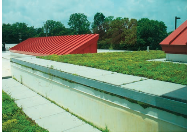
Figure 1: Greenroof on top of Hallsdale Powell Utility District, TN (Source: SMART Center).
