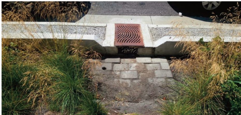
Figure 5.13: Paver inlet area of a bioretention cell that protects the media, dissipates inflow energy, and helps settle large solids for ease of maintenance.
