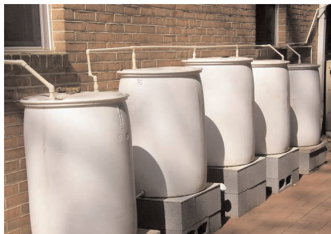
Figure 2: Set of rain barrels (Source: VADCR, 2011).
