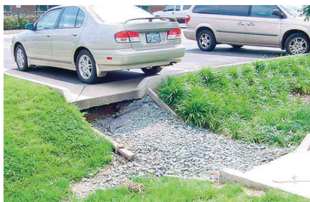
Curb inlets to bioretention swale have eroded because of improper sizing of stone.
