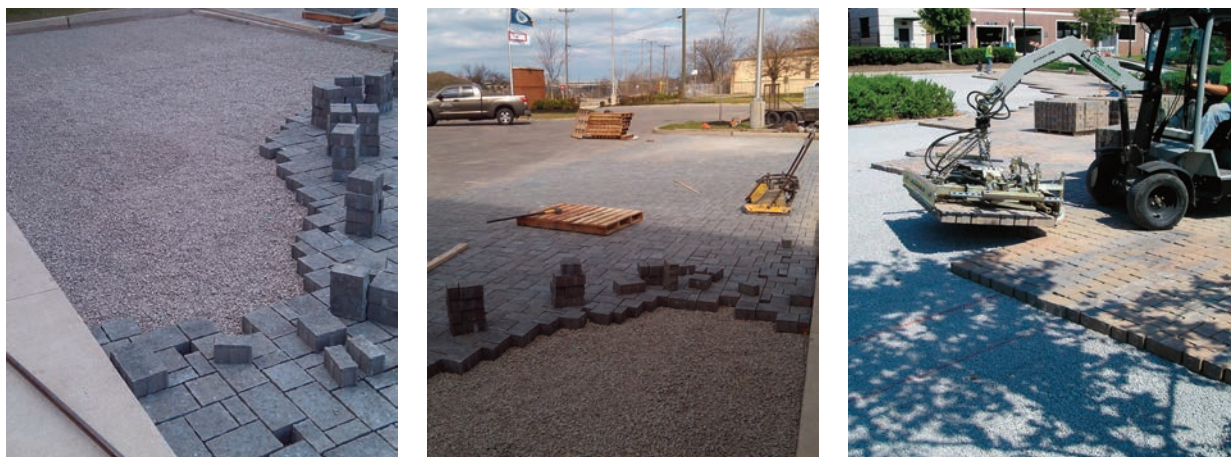
Figure 25: Alternative way of installing the permeable pavement (Source: R.K.).
