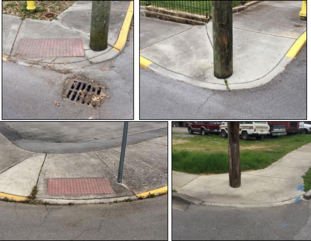
Examples of curb ramps with obstructions at turning spaces, on the ramp, or immediately adjacent to either.
