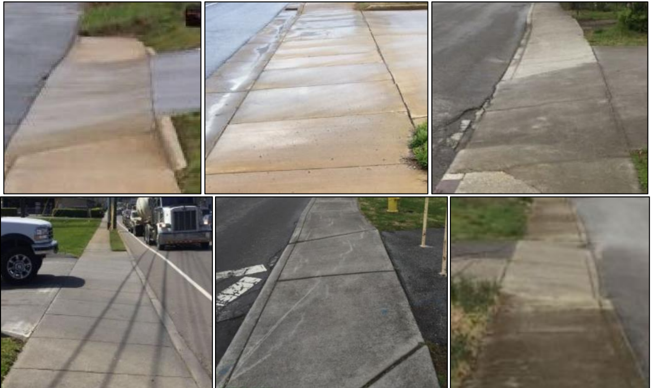
Examples of driveway transitions at the PAR that introduce severe cross slopes and/or vertical elevation changes.
