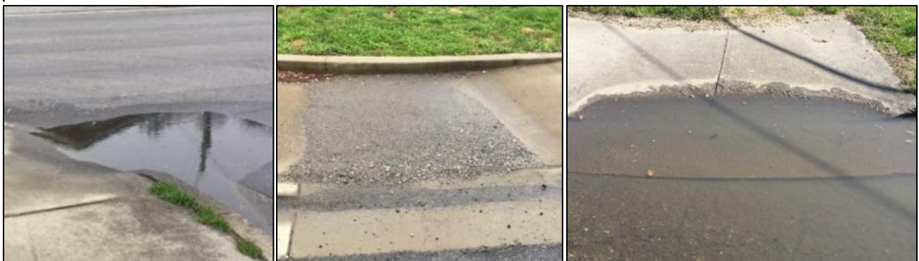
Examples of curb ramps with drainage issues and/or evidence of regular ponding, with sediment deposition.
