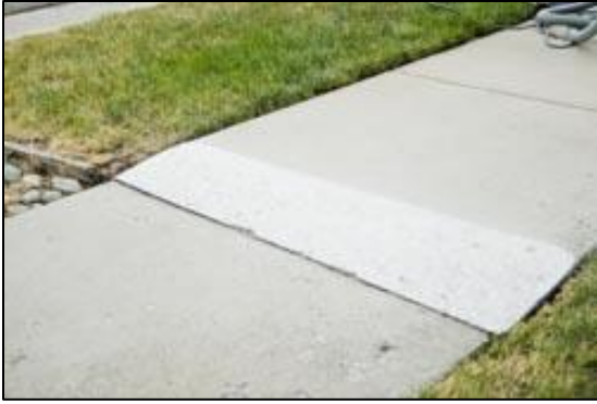
Grinding of small displacements
