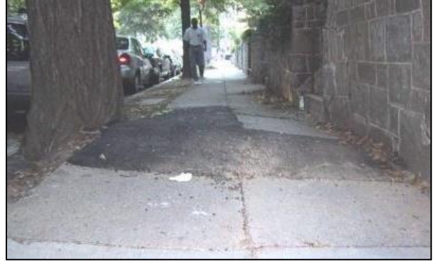
Temporary patching for large displacements
