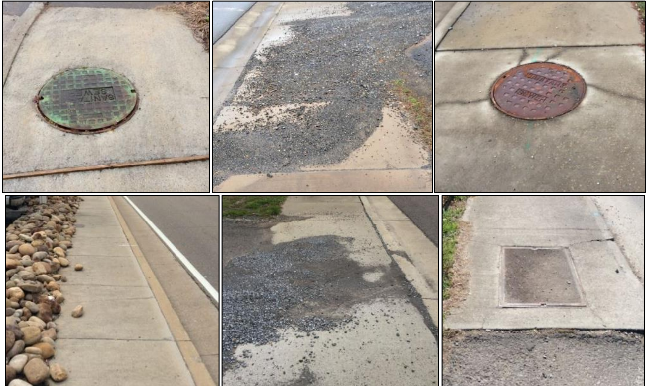
Examples of utility structures and debris along the PAR that can present issues for disabled users.
