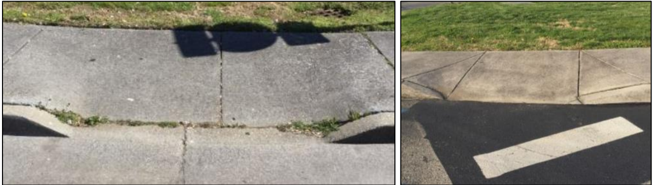
Example of curb ramps that have non-compliant flare slopes.
