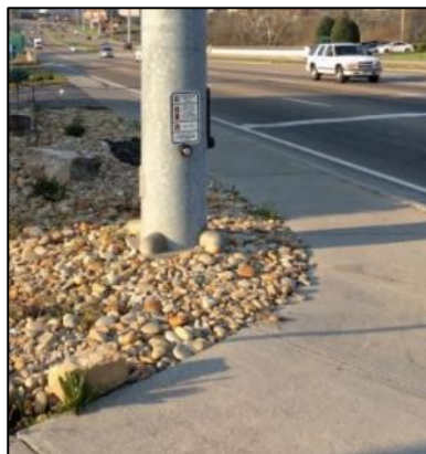
Example of pushbuttons that are not located on an accessible route.
