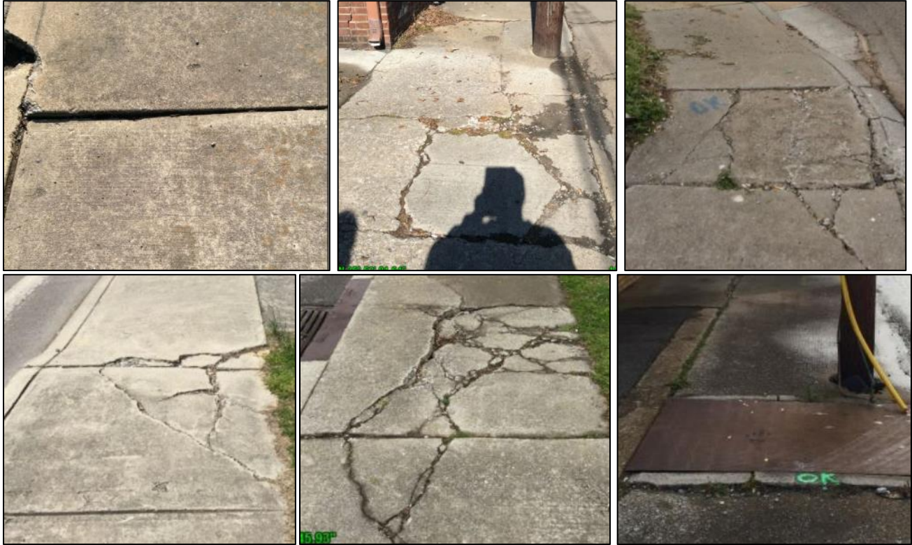
Examples of displacements, separations, and pavement in poor condition in need of maintenance.
