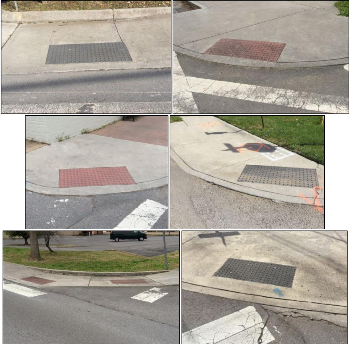
Example of curb ramps with detectable warnings that are not full width of the ramp.
