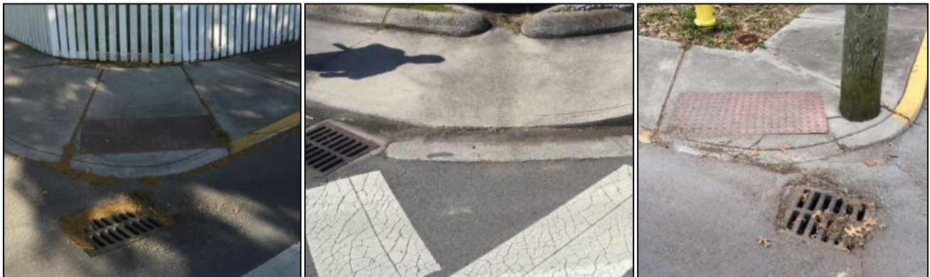
Examples of curb ramps with horizontal opening greater than \frac{1}{2} " on the ramp or the clear space.
