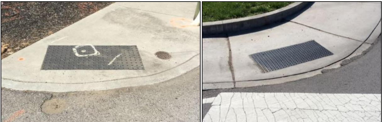
DWs that are oriented poorly and are not 24" depth in entire direction of pedestrian movement.
