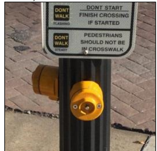
Example of non-compliant pushbutton operable parts (met previous standard)
