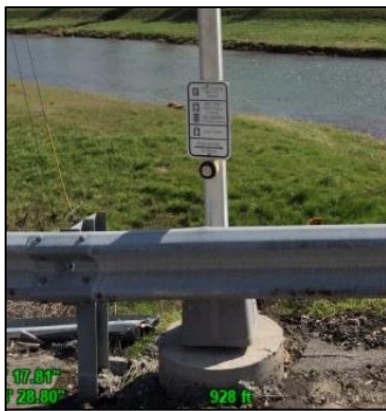
Example of pushbuttons that are not located on an accessible route.
