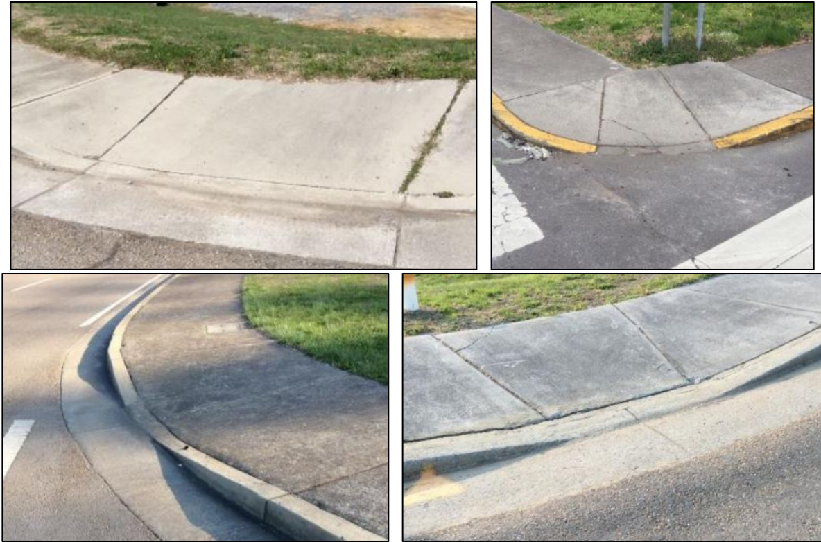
Example of curb ramps that lack a compliant turning space.
