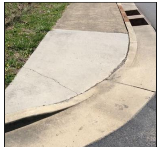
Example of curb ramp that does not provide the required perpendicular grade break.
