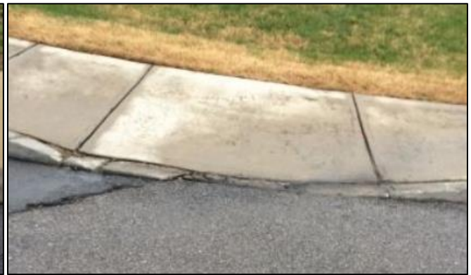
Curb ramps with excessive running slopes, typically severe slopes that exceed 10%. These ramps also exceed the counter slope requirements.
