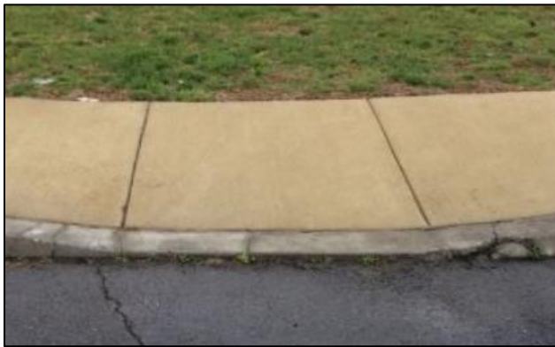
Curb ramps with excessive running slopes, typically severe slopes that exceed 10%. These ramps also exceed the counter slope requirements.
