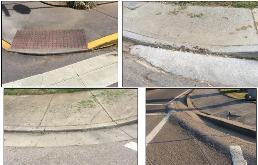
Examples of curb ramps with vertical discontinuities that exceed ½" at the curb, on the ramp, or the TS.
