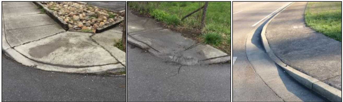
Examples of curb ramps that are less than the minimum 48" width required.
