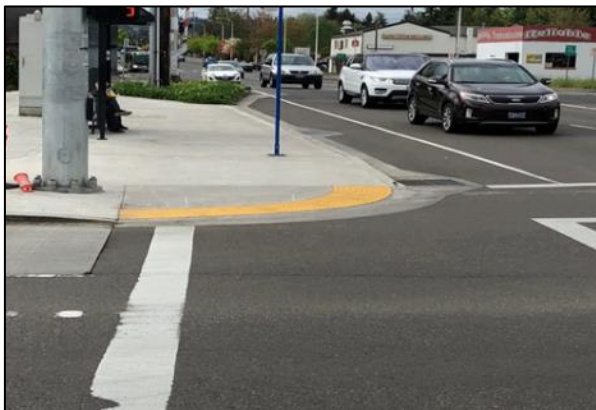
Diagonal blended transition (left) and diagonal perpendicular ramp (right). Both provide access to street crossings of more than one direction and are no longer permitted by PROWAG per R207.1.
