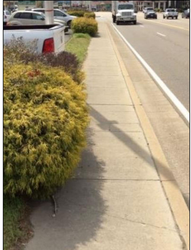
Example of overgrown vegetation that reduces the PAR width to less than 48".
