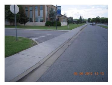
On sections of streets equipped with a separate greenway section, the driveway entrance shall be constructed of 6" minimum thickness concrete through the entire width of the greenway section. Greenway shall be connected with the driveway entrance in accordance with ADA standards. See example below:
