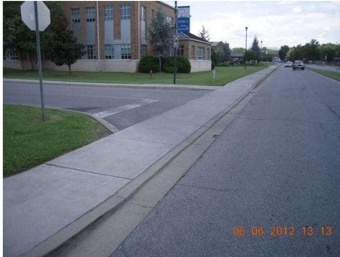
On sections of streets equipped with a separate greenway section, the driveway entrance shall be constructed of 6" minimum thickness concrete through the entire width of the greenway section. Greenway shall be connected with the driveway entrance in accordance with ADA standards. See example below:
